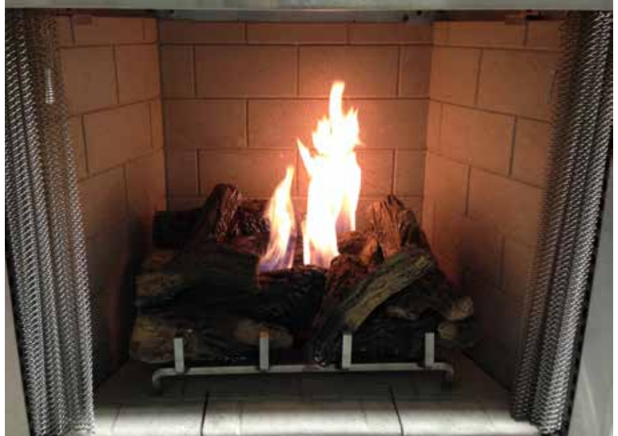
Figure 23 - Proper Burner Flame Appearance
